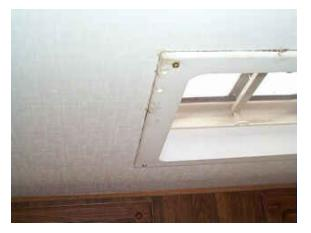
A leak in the ceiling usually shows up on the inside of the coach some time after the initial leak. Often, long after the leak has occurred! In that case, there will likely be some dry rot damage to the wooden roof structural members.
