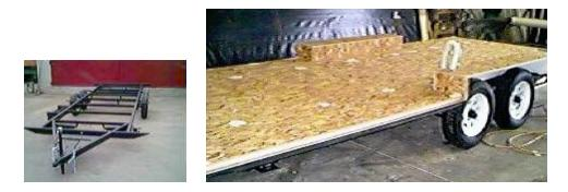
Upon this platform, the floor is laid, with the lino and carpet installed, and the interior appliances, cabinets, and interior partitions are fastened directly to the floor through the finished flooring material. Next the walls are put on as complete units or ready to have the siding installed, depending on the construction method. Finally, the roof is laid onto the top of the walls and is fastened to them and to the top structures of interior cabinets.
