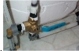
Single valve in bypass position.
