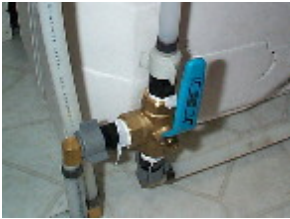
Single valve bypass in the normal flow position.
